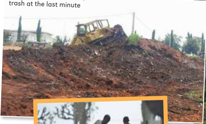
The digger cleaning out piles of trash at the last minute
